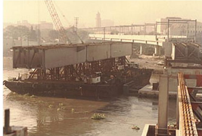
Figure 1. Construction of LRT 1
